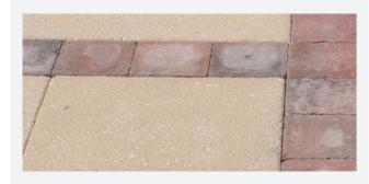
Efflorescence is an unpredictable, but temporary, process. Once all the salt from the paving has risen to the surface it is commonly worn away through use or by weathering. This process seldom takes more than 12 months.
